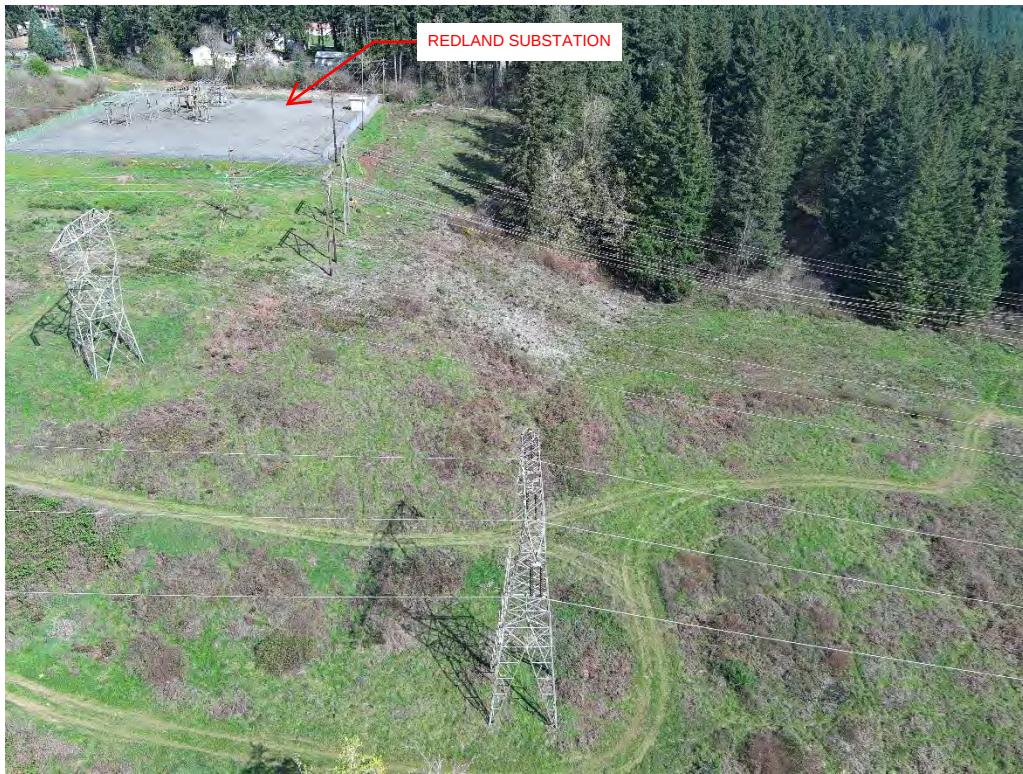
PHOTOGRAPH 2: VIEW OF MAPPED DOGAMI LANDSLIDE AREA, LOOKING NORTH
