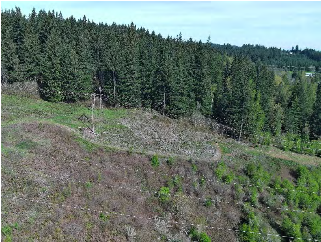
PHOTOGRAPH 3: VIEW OF INFERRED LANDSLIDE AREA, LOOKING NORTH
