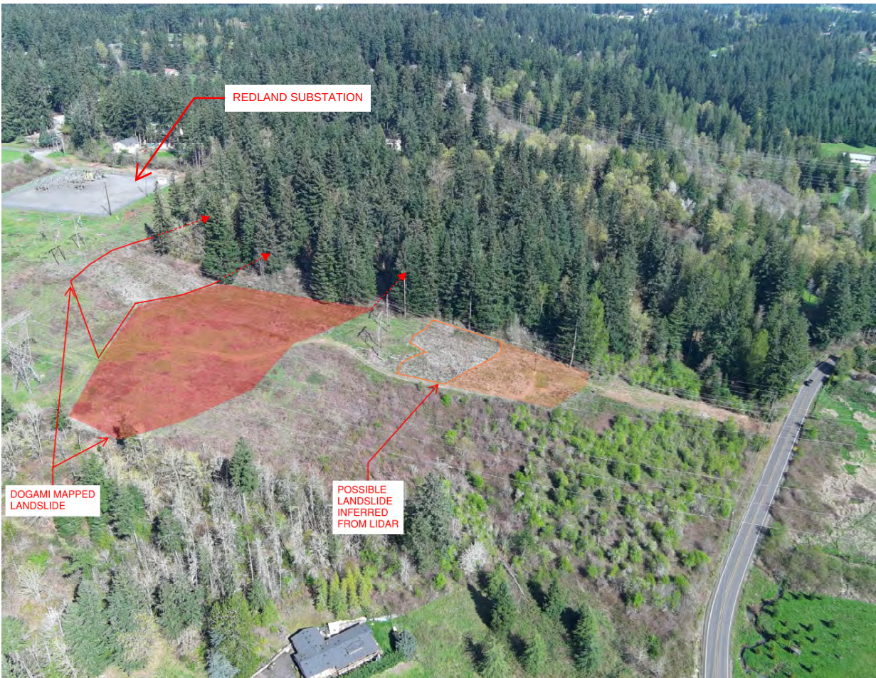
PHOTOGRAPH 1: SITE OVERVIEW LOOKING NORTH. DASHED LINES AND ARROWS SHOW WHERE MAPPED DOGAMI LANDSLIDE CONTINUES NORTH OF THE TRANSMISSION LINE CORRIDOR
