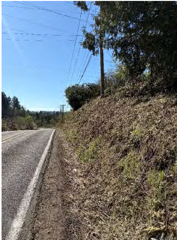
PHOTOGRAPH 4: VIEW OF S HENRICI ROAD CUT, LOOKING SOUTHWEST
