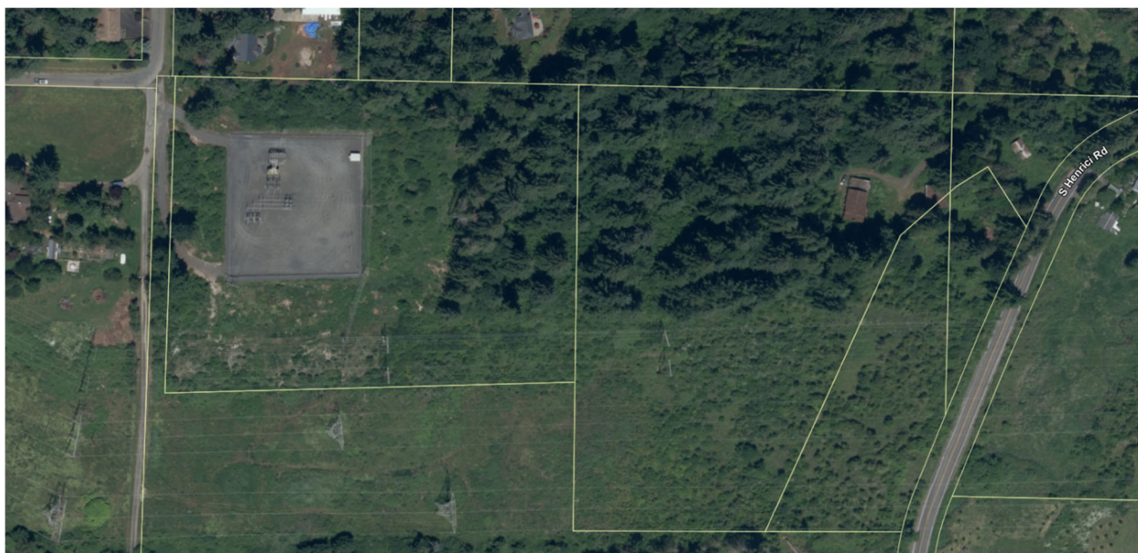
Figure 1. Aerial Photo of Redland Substation
