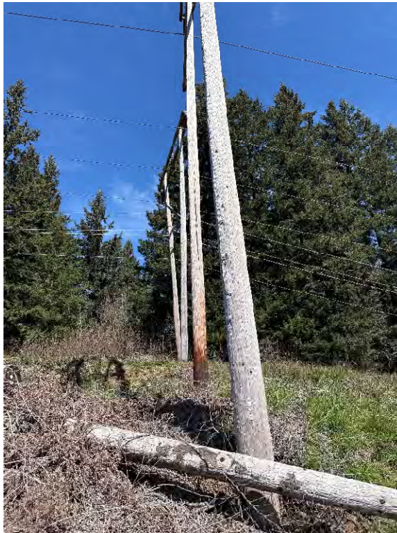
PHOTOGRAPH 5: VIEW OF POLES 2157/2158 AND 2159/2160, LOOKING NORTH
