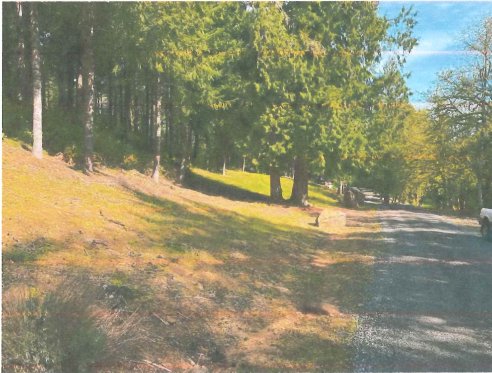
Photo 2 View looking downslope toward access road showing gently to moderately sloping terrain with grass cover, scattered trees, and localized exposed soils. Slope appears uniform and stable with no evidence of active erosion or slope distress
